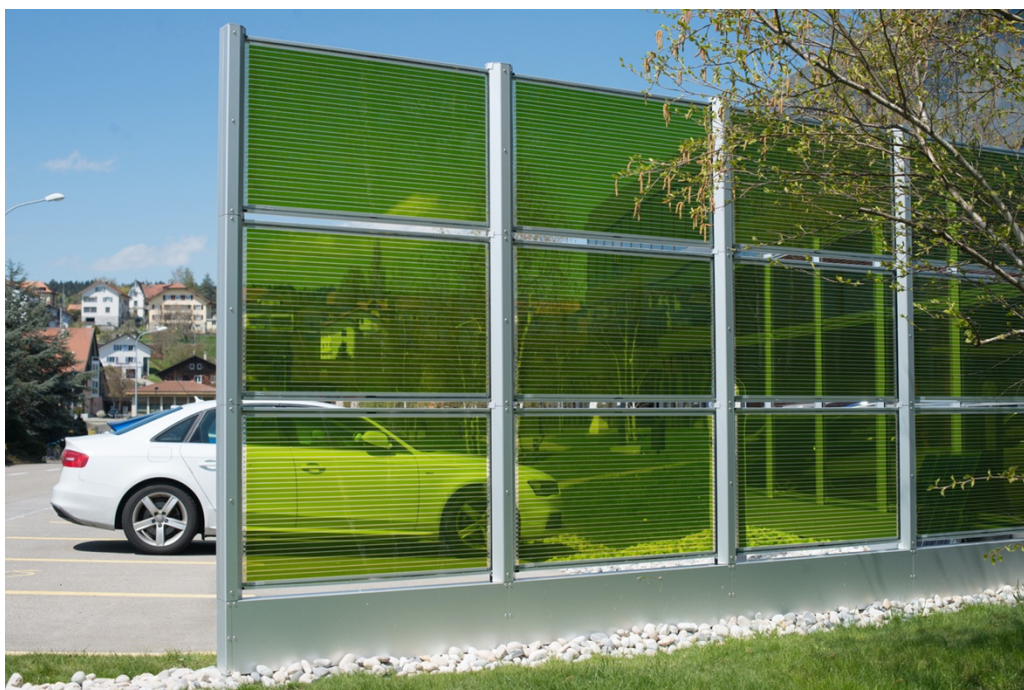
Figure 1 Electric car charging statio, powered by dye sensitized solar cell panels near Villa-Saint-Pierre, Switzerland.
